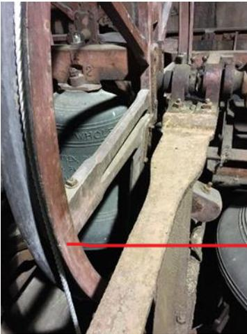
In this picture you can see a typical bell frame and bell wheel. The bells are in the down position and we can see that we can easily mount the transmitter on the horizontal frame
